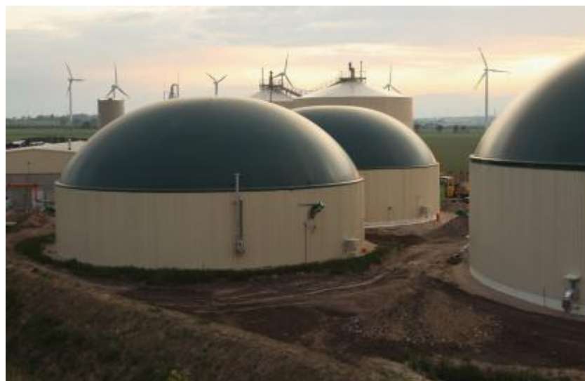
Figure 131: Wind turbines near a new biogas plant in the German state of Lower Saxony 3
