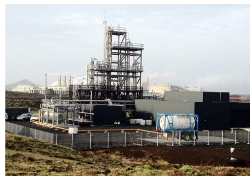
Figure 147: George Olah renewable methanol plant, Svartsengi, Iceland
