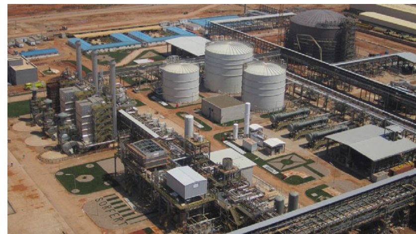
Figure 186: Greenfield fertilizer plant of Sorfert Algeria built by Orascom Construction Group 1
