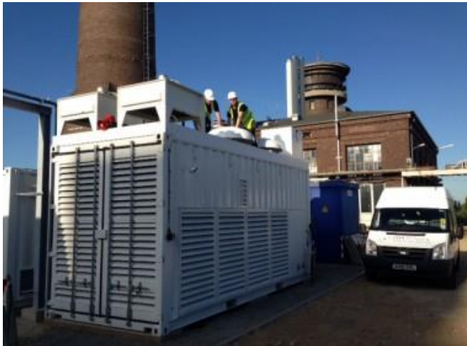
Figure 200: Thüga Group power-to-gas electrolyzer plant (left) and layout (right)
