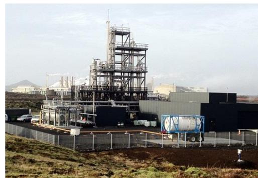
The 2.8 MW<sub>ch</sub> Carbon Recycling International plant started operating in late 2011. It uses cheap geothermal electricity and CO<sub>2</sub>, sourced from the nearby HS Orka geothermal power plant. Methanol is sold as a renewable fuel under the name Vulcanol, to be mixed with gasoline. CRI plans to scale up the technology, with 30 MW<sub>ch</sub> plants across the world.
